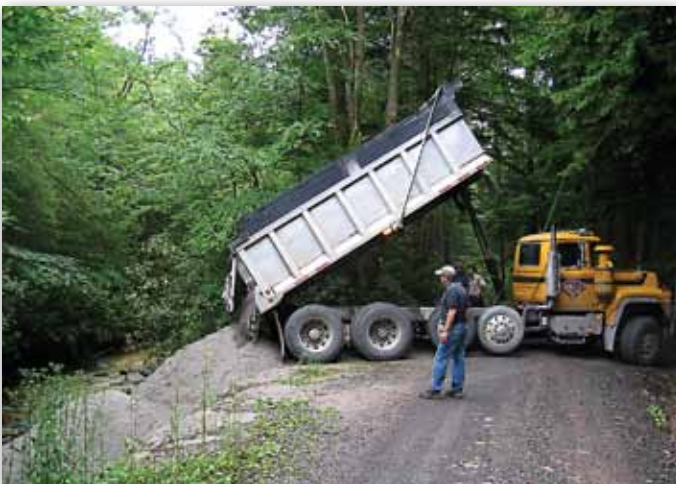
Limestone sands dumped into tributaries of the Cheat River help neutralize acidic waters in the stream and in the lake downstream.
